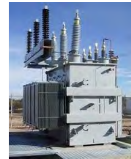
Station Class Transformer Refurbs
