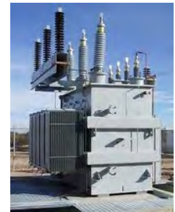
Station Class Transformer Refurbs
