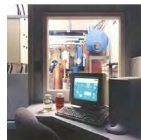
Plant Control Room
